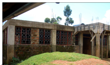
Progress on the three-story building
